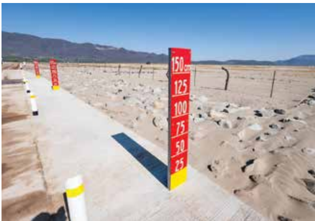
Spillway and flood level signs at a wetland restoration area.
